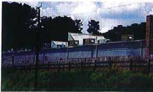
This is not adequate screening or detailing
