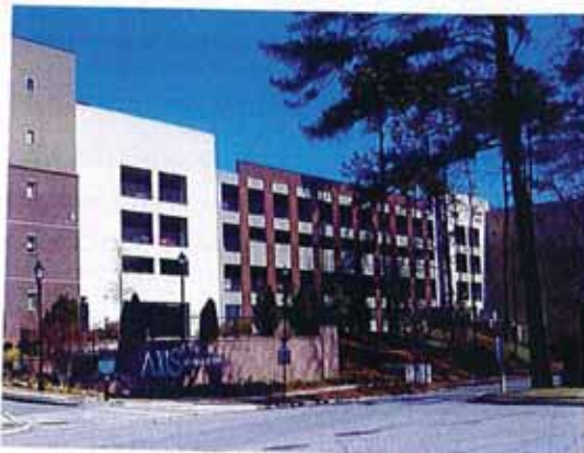
Below: not acceptable design of a parking structure.
