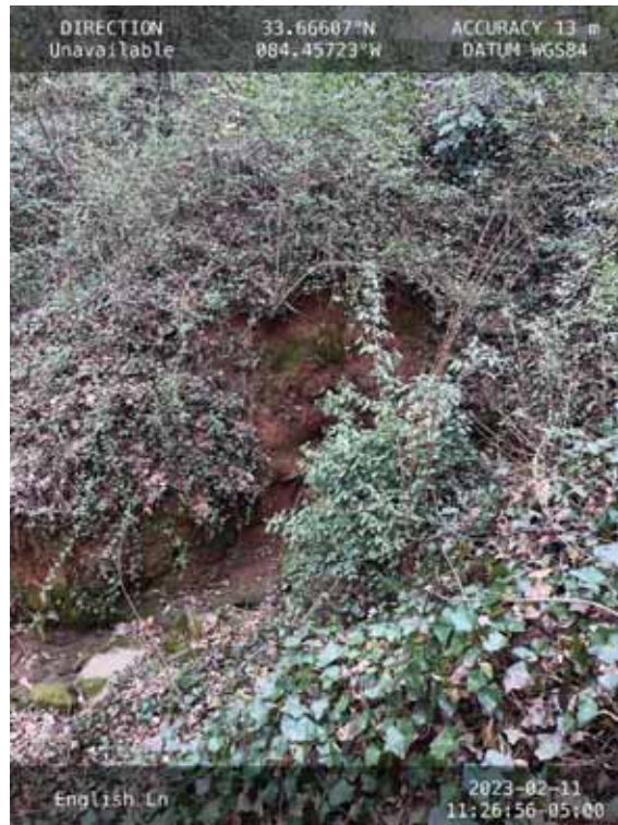
Down-cut gully as the channel enters the property.
